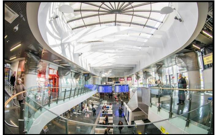
Transparent polycarbonate used in previous constructions was replaced by tempered greyish blue glass. Lighting of the check-in hall and entries, over which illuminated inscriptions appeared, is ensured by LED strips and luminaires. Renovated at the expense of PLN 1.4 million, a part of the underground passage was opened at the turn of 2015 and 2016.
